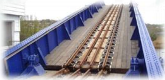
Photos of Bann Bridge being raised, vessel movement through bridge and existing fendering system
