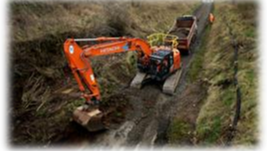
Track Dig Out Formation
