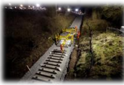
Placement of Sleepers and Rail
