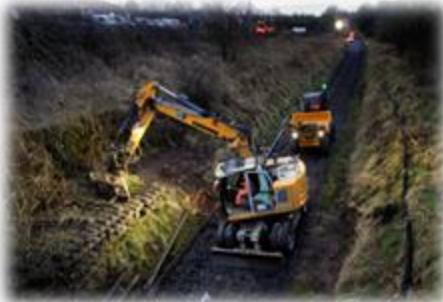
Removal of Rail and Sleepers
