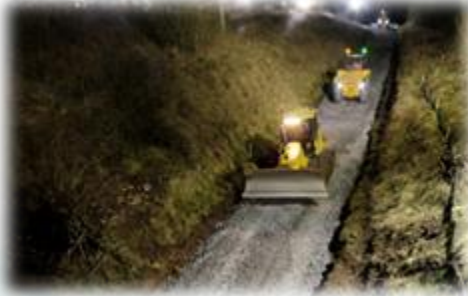
Bottom Ballast Placed and Rolled
